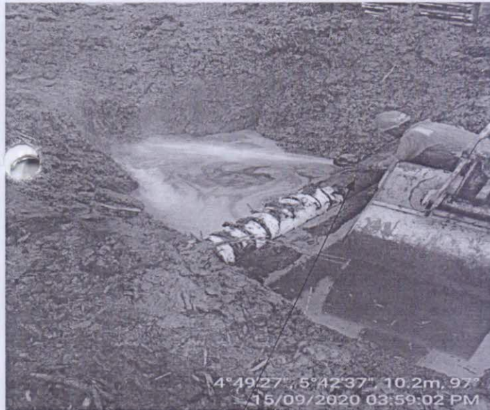
UNWRAPPING THE PIPELINE FOR SPILLED POINT ASSESSMENT BY THE REPAIR PERSONNEL
